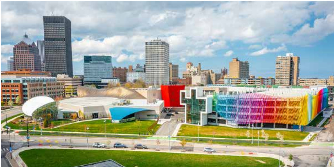
Museum and Parking Garage Exteriors
